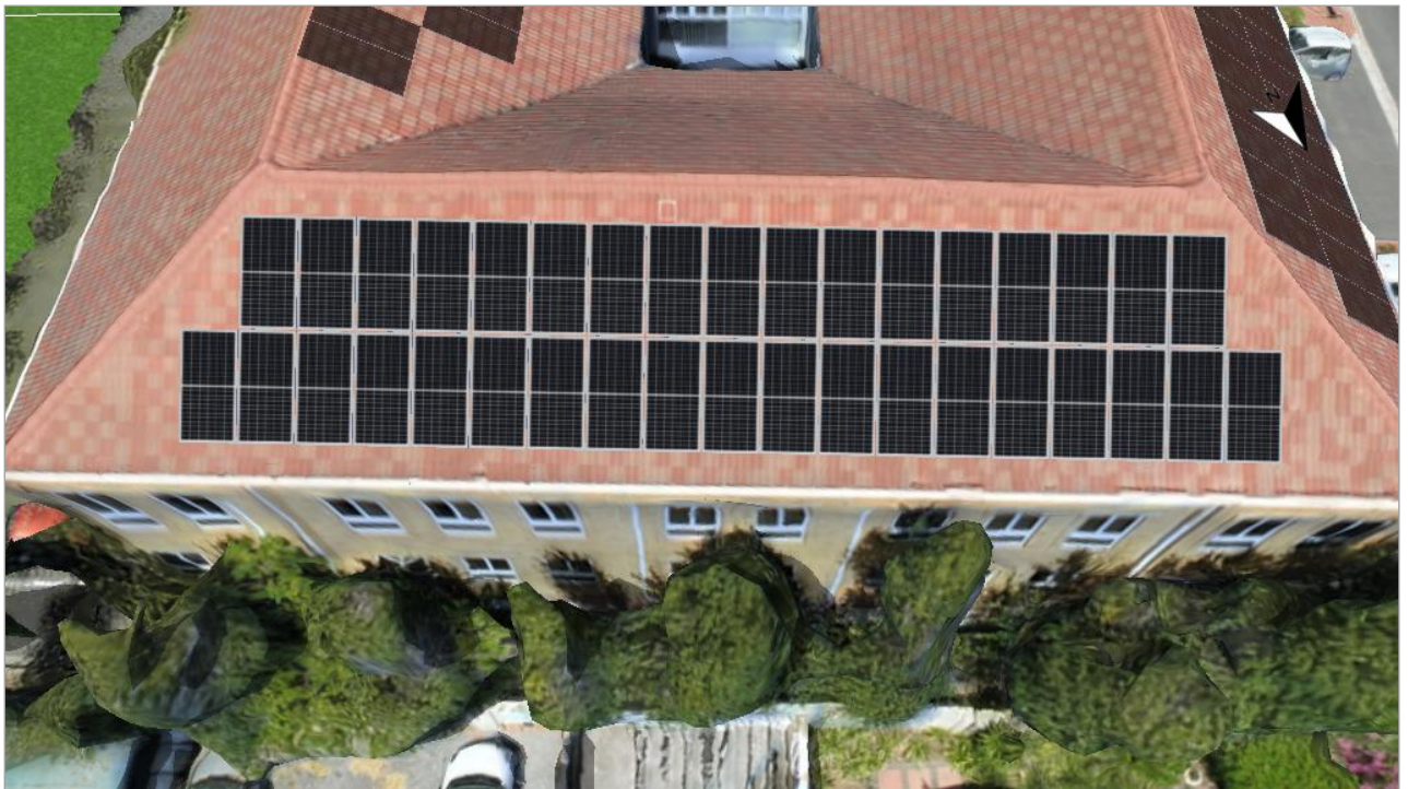
Figure: 1. Module Area - TrizEng 01-North EAST1
